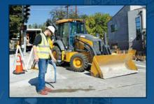
**Interference** is an electrical disturbance that can affect the accuracy of the locator, typically caused by substations and buried or overhead high voltage cables
